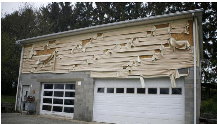
House “B” was 800’ away from the breach. It was so hot that the vinyl siding melted from the garage.
